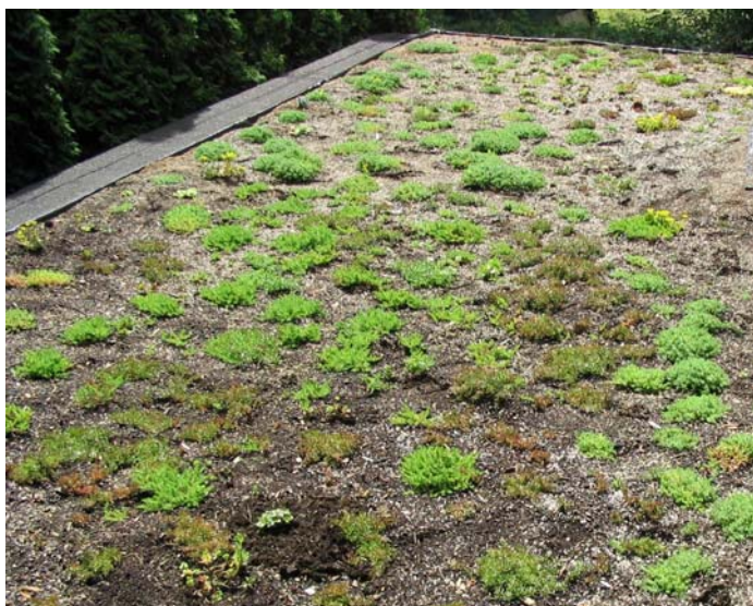
Guild member Jon Alexander's sedum planted green roof, one month after planting. Jon's roof also contains raised beds for vegetable gardening.
