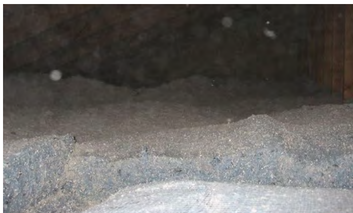
Any attic insulation should be smooth across the entire home. Mounding, lumps, valleys, voids and other problems with uniformity significantly reduce the overall R-value of the insulation. Source: O'Brien360
