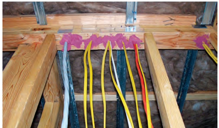
In an addition, new construction or a gut remodel, there are many opportunities to seal electrical penetrations and top and bottom plates. Source: O'Brien360
