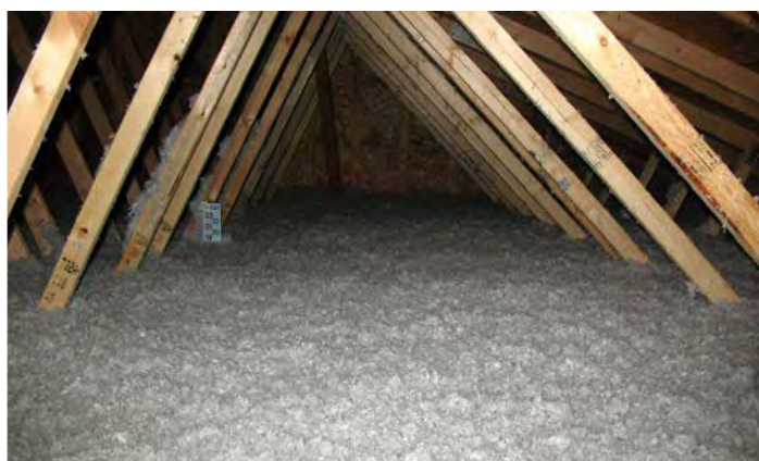
Here, loose-fill blown cellulose insulation covers the attic correctly – there is no indication of more or less insulation in any one area. Depth is uniform and smooth, and the code-required insulation ruler is visible near the back left to demonstrate insulation depth. Source: O'Brien360
