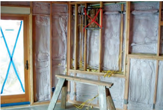
This picture shows the "flash" portion of a "flash and batt" installation. The flash coat of spray-in-place foam insulation creates a tight air seal. Source: O'Brien360
