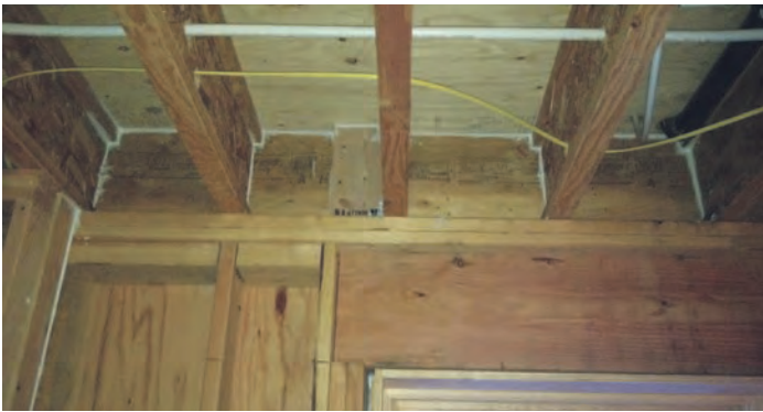
Air sealing with expanding foam or caulk at a rim joist is an effective means of sealing leaks. Source: O'Brien360
