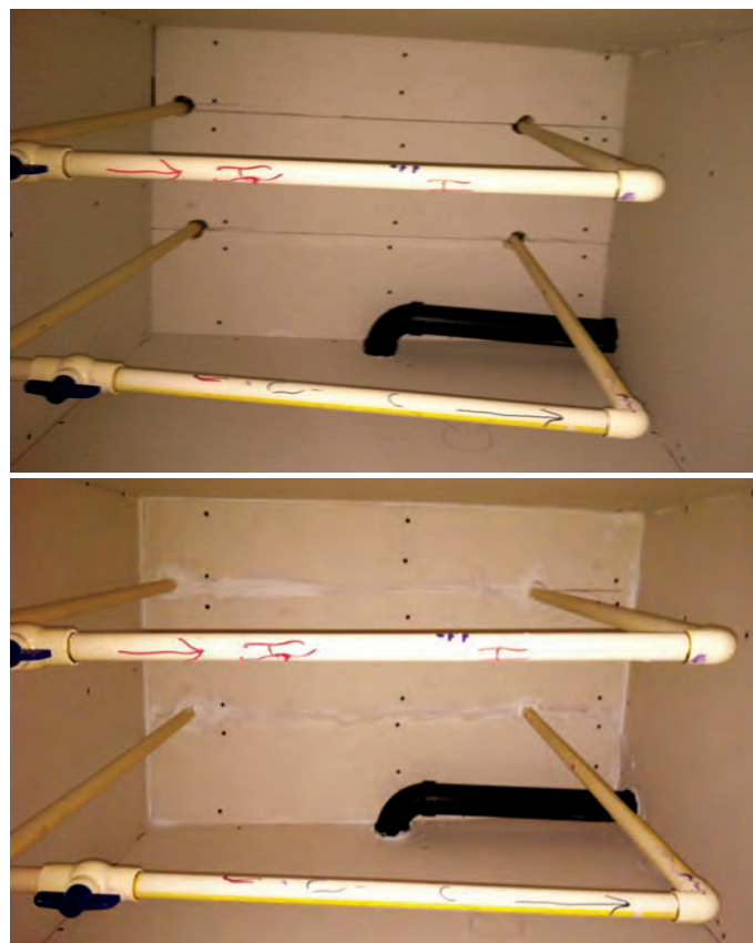
These pictures show before and after air sealing efforts at plumbing penetrations. Source: O'Brien360.
