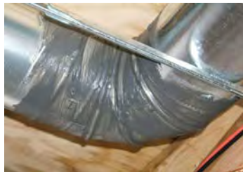
This metal duct elbow seam with properly sealed with duct mastic. If the ducts are in the crawl space, attic, or garage, they should be insulated after being well sealed. Source: O'Brien360
