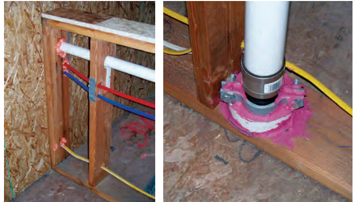
In a kitchen or bathroom remodel, or new construction, sealing plumbing penetrations is easy and effective. Source: O'Brien360
